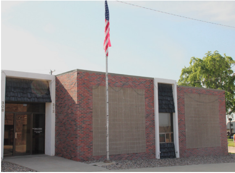
First National Northeast Hartington
