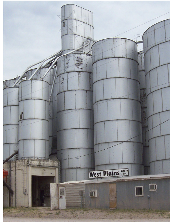
West Plains Grain Elevator - Crawford
