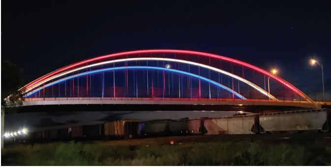
33rd Avenue Viaduct
