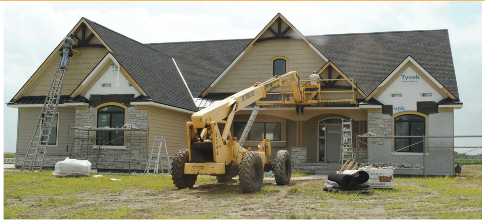
New home construction
