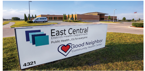
East Central District Health Department & Good Neighbor Community Health Center
