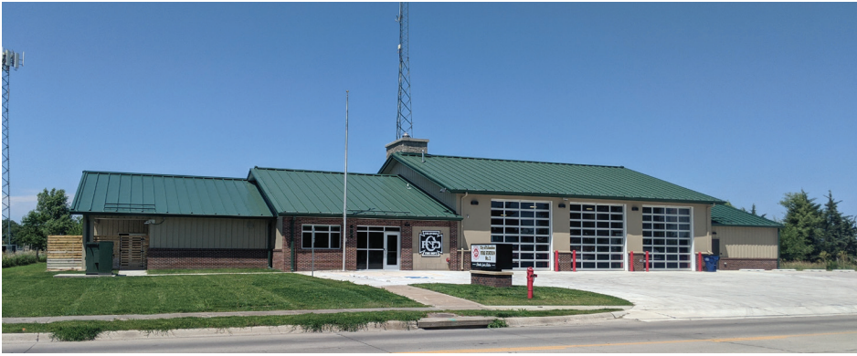
Columbus Fire Station #2
