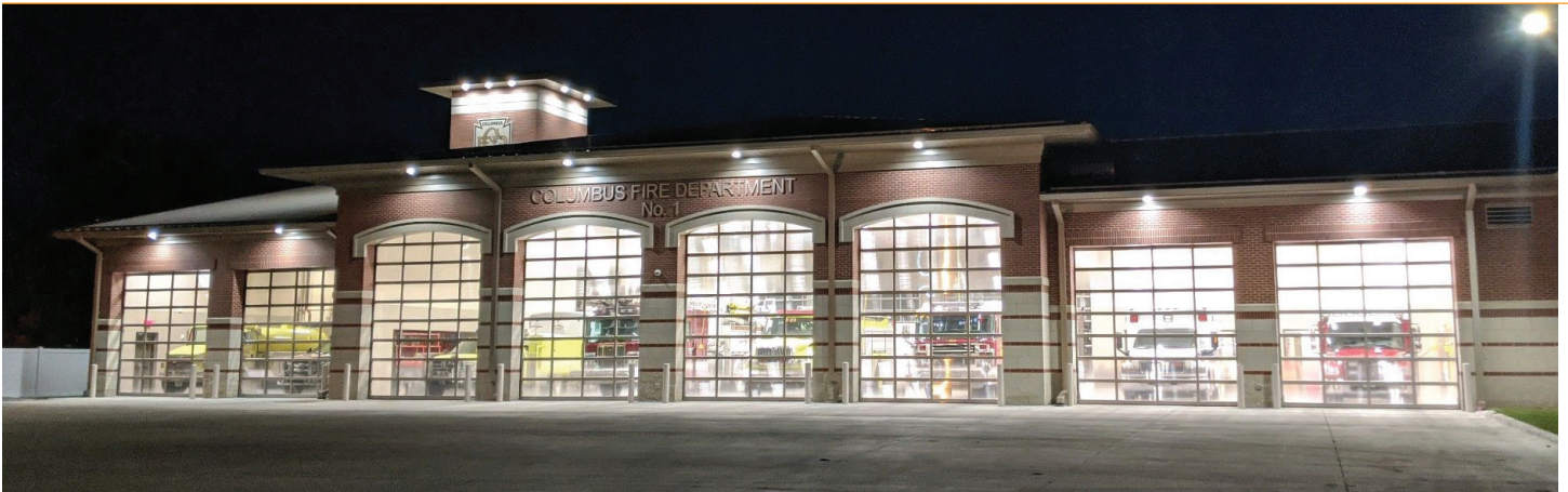
Columbus Fire Station #1
