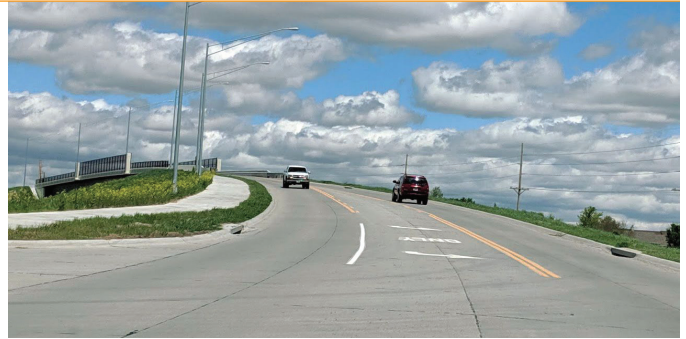
3rd Avenue Viaduct
